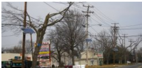
Solar panels on power poles, New Jersey
